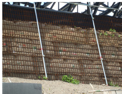
LandscapeCL is ideal for embankments
